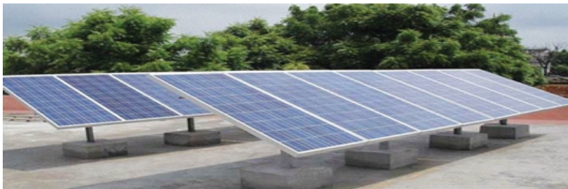
2.24 kW SPV Power Plant at Panchayat Samiti, Dudu, Distt. Jaipur, Rajasthan, Source: mnre.gov.in
