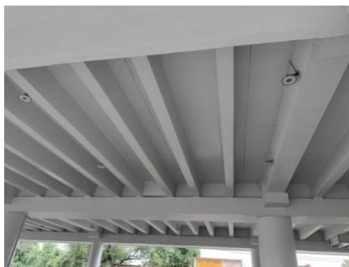
Photo 5(a): Double-T Girder used at IIT Kanpur Metro Station. (b) The envoy with Project Director Er. Arvind Singh
