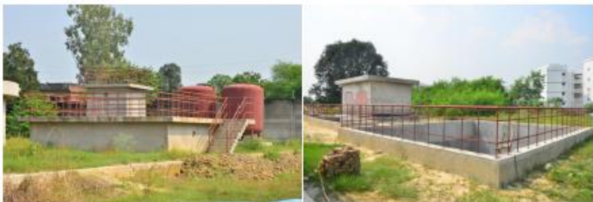
Figure 3.3: Sewage Treatment Plant
