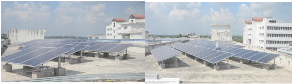
Figure 4.3: Solar light installation on the terrace of Departments.
